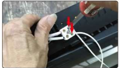
F: fix the two wires inside and screw them
